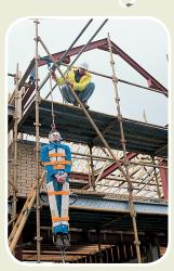
Vertical lift using integral lifting O-ring and foot-end guide rope
